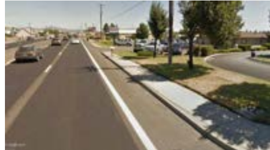
Figure 8: Typical curb-tight sidewalk condition
