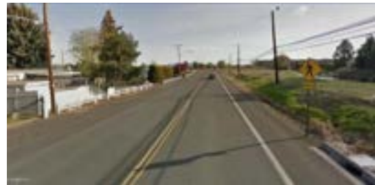
Figure 10: Canal Blvd lacks continuous sidewalks
