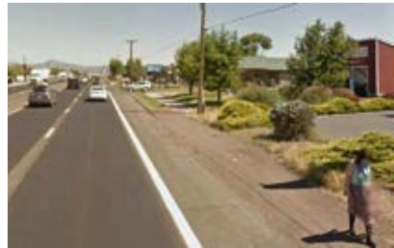
Figure 5: Frequent sidewalk gaps along US 97
